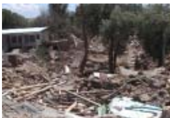
The building completely destroyed by the earthquake, Cahngoureh, near the epicenter
