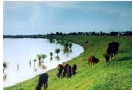
The land in low-lying areas of the river delta is protected against flooding by river dyke systems. According to official historical records, in 1108, King Ly Nhan Tong ordered the construction of the first dyke with solid foundations on a large scale aimed at protecting the capital of Thang Long (now Hanoi). For years, the dyke has been upgraded and considered a symbol of the Vietnamese people's strong will and vitality.
