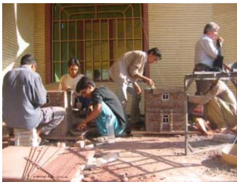
Figure 1: Local masons at on-the-job-training for earthquake resistant construction
