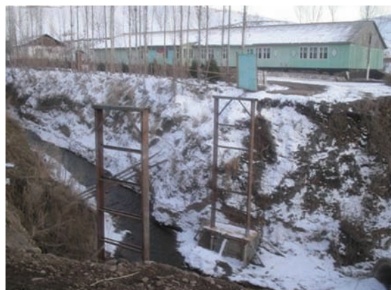
Start of mitigation
