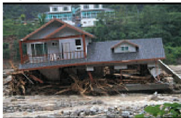
Flood Damage by Torrential Rain in 2006
