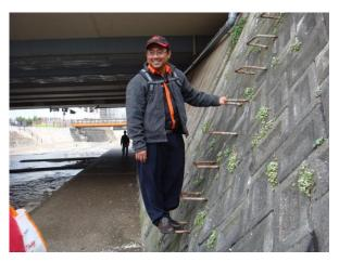
Fig. 4-1-7 Evacuation ladder along the Toga River, Kobe.
