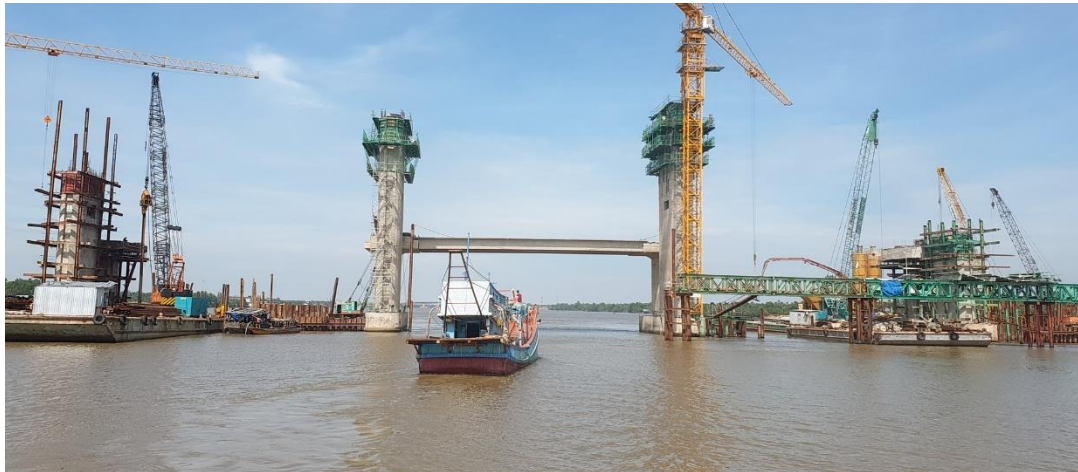
Figure 19 : Cai Lon – Cai Be irrigation system under construction
