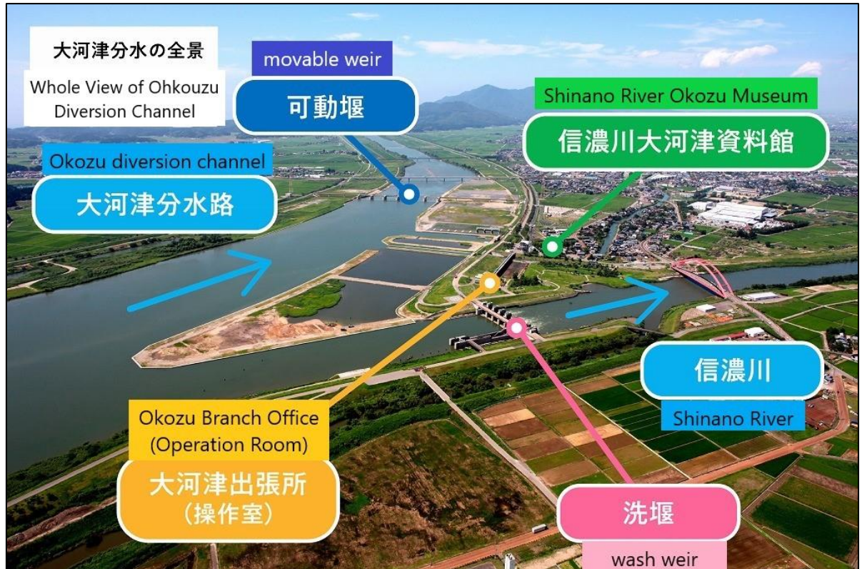
Figure 11 : Whole View of Ohkouzu Diversion Channel
