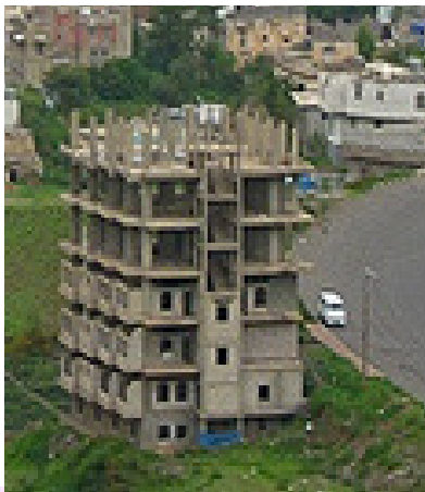
Concrete Filled by block
