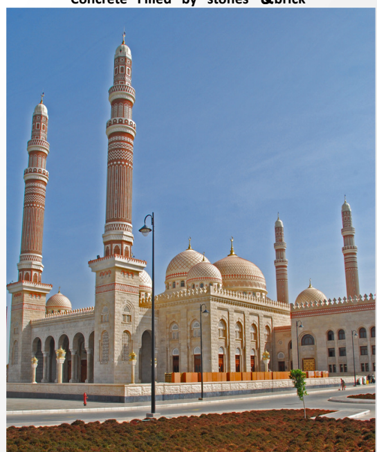
Concrete Filled by stones & brick
