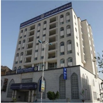
Concrete Filled by Heavy stones
