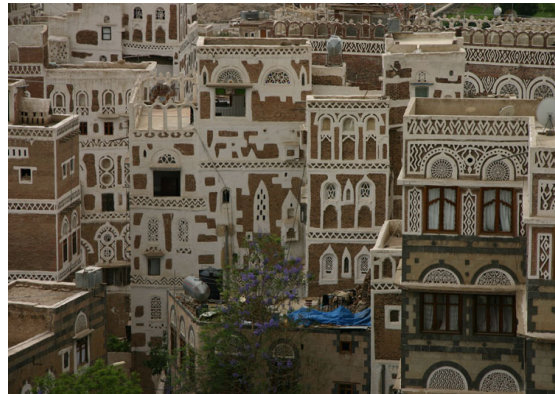
Burnt Brick + stone
