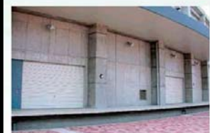
Truck yard (for transporting supplies)
