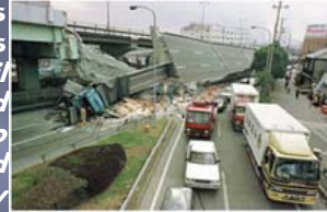
A truck fallen from collapsed Iwaya overhead bridge of national road 43
