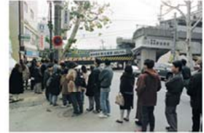
A collapsed overhead railroad near the Shinzaikai Station of Hanshin Railway
