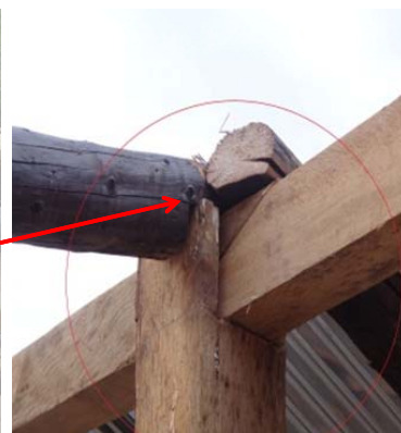
Failure at roof ridge connections
