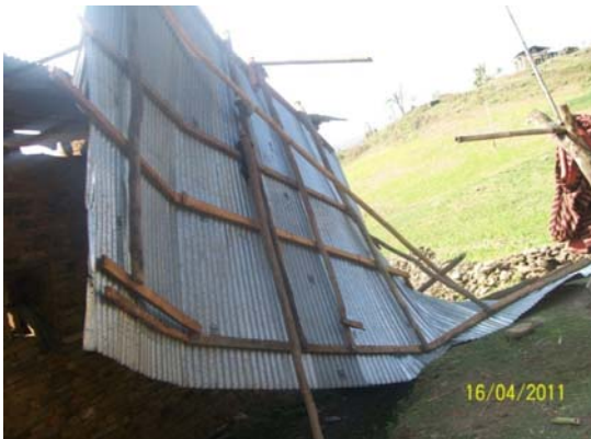
CGI sheet lift/loss at roof edges and gable roof end
