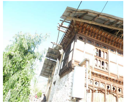
CGI sheet lift/loss at roof edges and gable roof end
