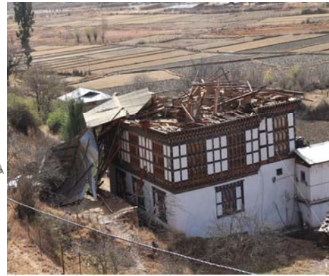
Full blown-off or overturning of roof failure
