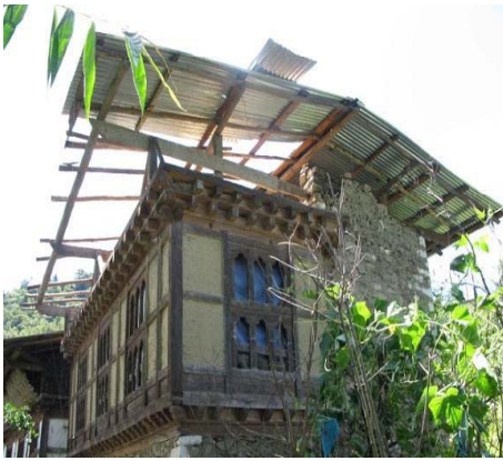
CGI sheet lift/loss at roof edges and gable roof end
