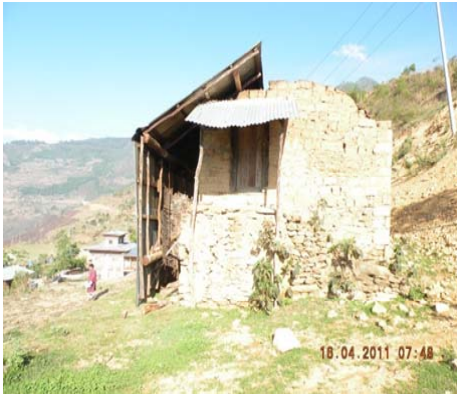
Full blown-off or overturning of roof failure
