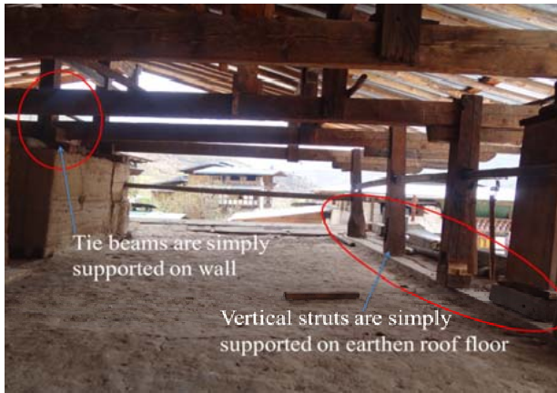
Full blown-off or overturning of roof failure
