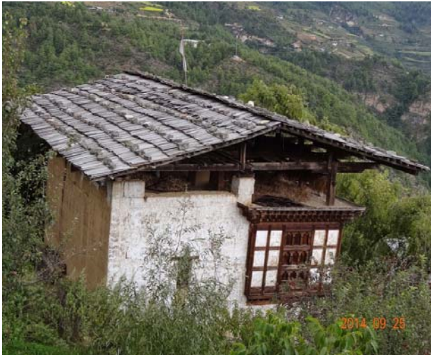
Hip-and-gable roof with CGI sheets
