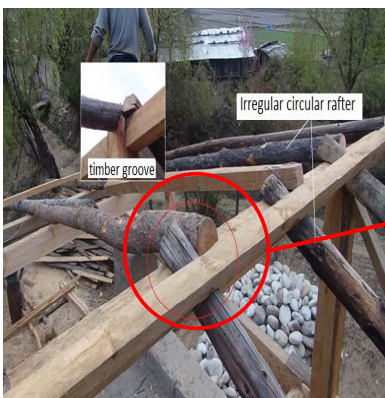
Failure at roof ridge connections
