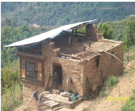
Failure at roof ridge connections
