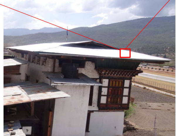
Hip-and-gable roof with CGI sheets
