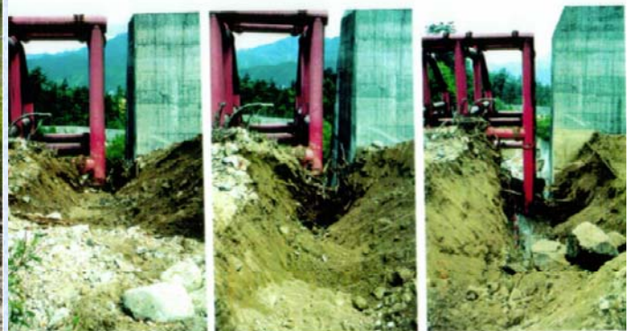
Grid Sabo dam with trapped debris flow
