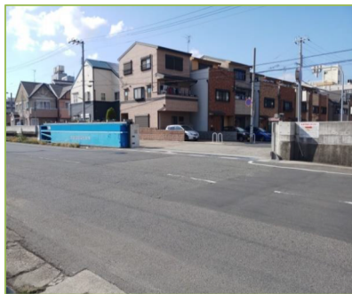
Flood gate at Higashi-nada ward in Kobe
