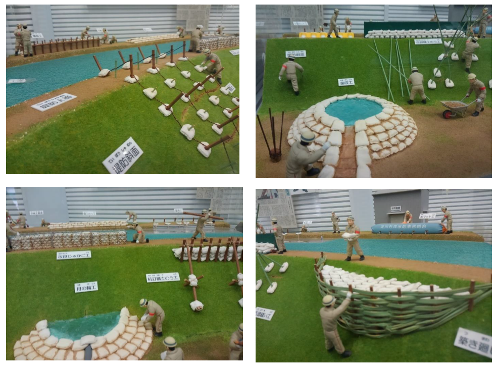
Models showing activities on Flood Protection/ Prevention by Suibo-Dan (Flood Fighters) using sand bags, bamboo and local materials (photo source: Tsunami & Storm Surge Disaster Prevention center, Osaka)
