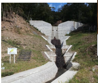
Sabo works for sediment erosion control in Tamba city
