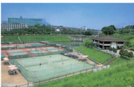
Kirigaike regulating reservoir, Kanagawa Prefecture This is normally used as a tennis court.
