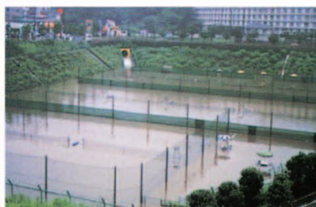
Reservoir filled with water in June 1985
