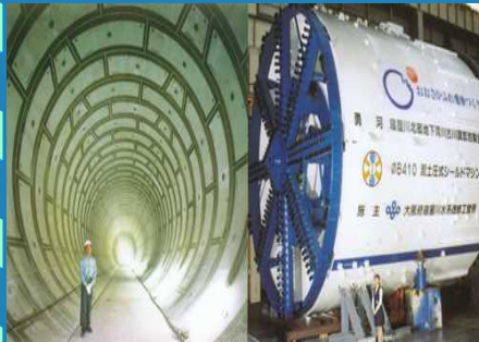
Neya river northern section underground flow
