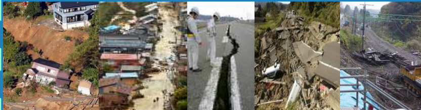
Cause to many huge landslide, flood and mudslide, damaged roads & railways
