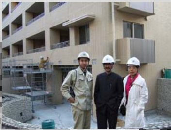
Construction Site Sannomiya
