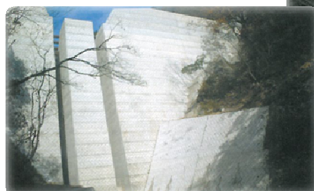
Completed reinforced dams
