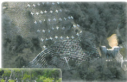
Grating crib works preserving existing vegetation (slope stabilization)
