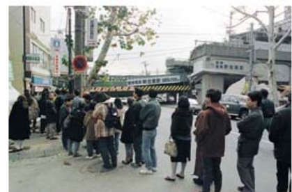
A collapsed overhead railroad near the Shinzaike Station of Hanshin Railway
