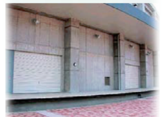
Truck yard (for transporting supplies)
