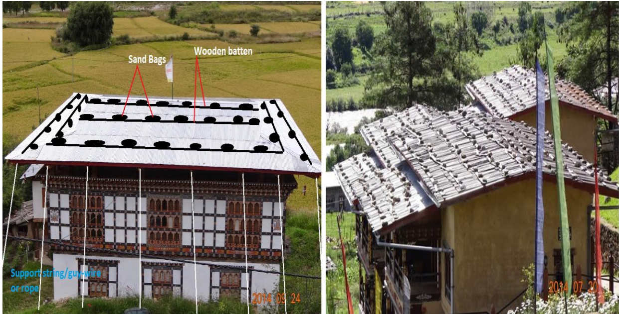
Figure 61: Support string or guy-wire or rope and sand bags (L) and wooden shingle over CGI sheet metal with stone (R)
