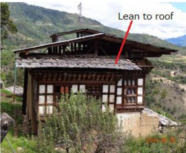
Figure 8 : Lean-to roof with shingle roofing (L) and CGI sheet roofing (R)
