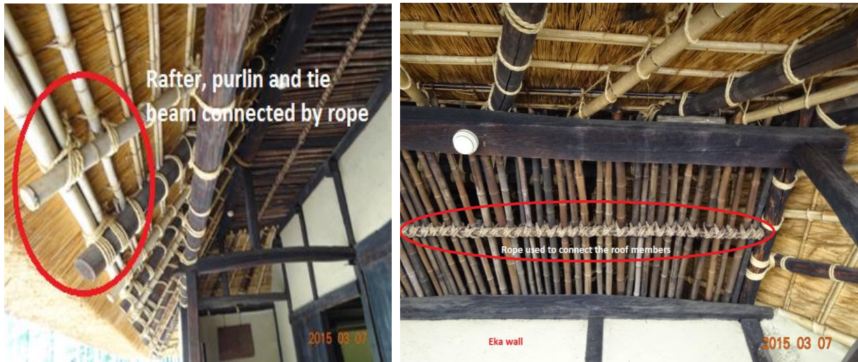
Figure 58: Japanese thatched roof connection using ropes
