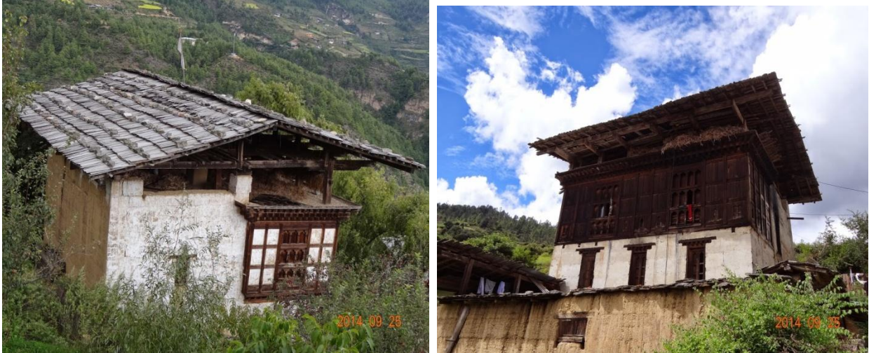
Figure 2: Traditional Bhutanese gable roof with shingle roofing
