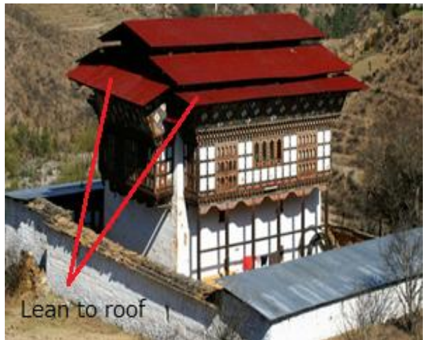
Figure 8 : Lean-to roof with shingle roofing (L) and CGI sheet roofing (R)
