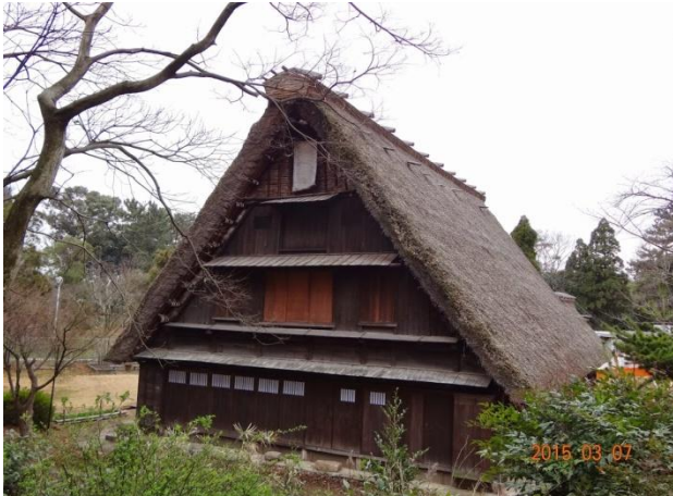
Figure 21 : Gable roof (kirizuma) with thatched roofing (L) and cryptomeria bark roofing (R)
