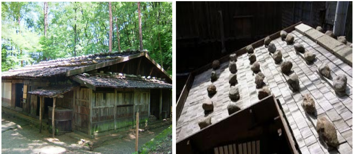
Figure 27: Shingle or plank roofing in Sado Island Niigata (photo courtesy: Brian Southwick)
