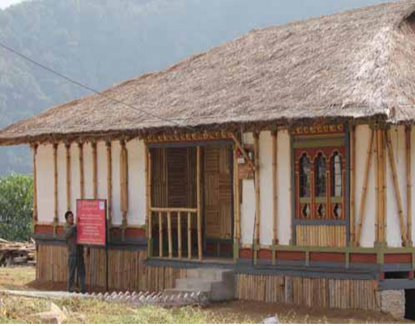
Figure 10 : Thatched roofing (L) and bamboo mat (R)
