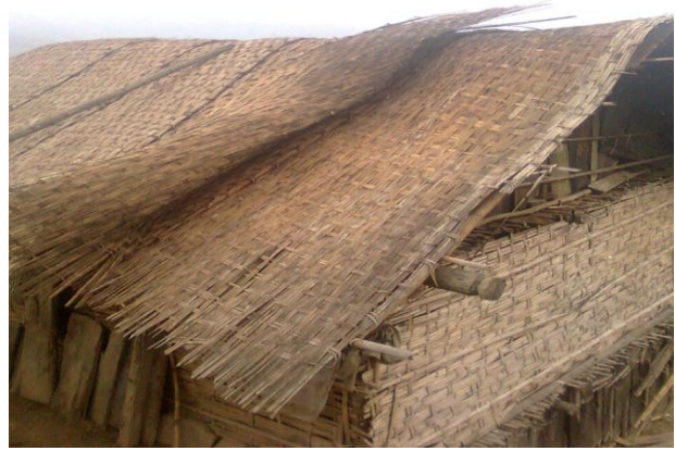
Figure 10 : Thatched roofing (L) and bamboo mat (R)
