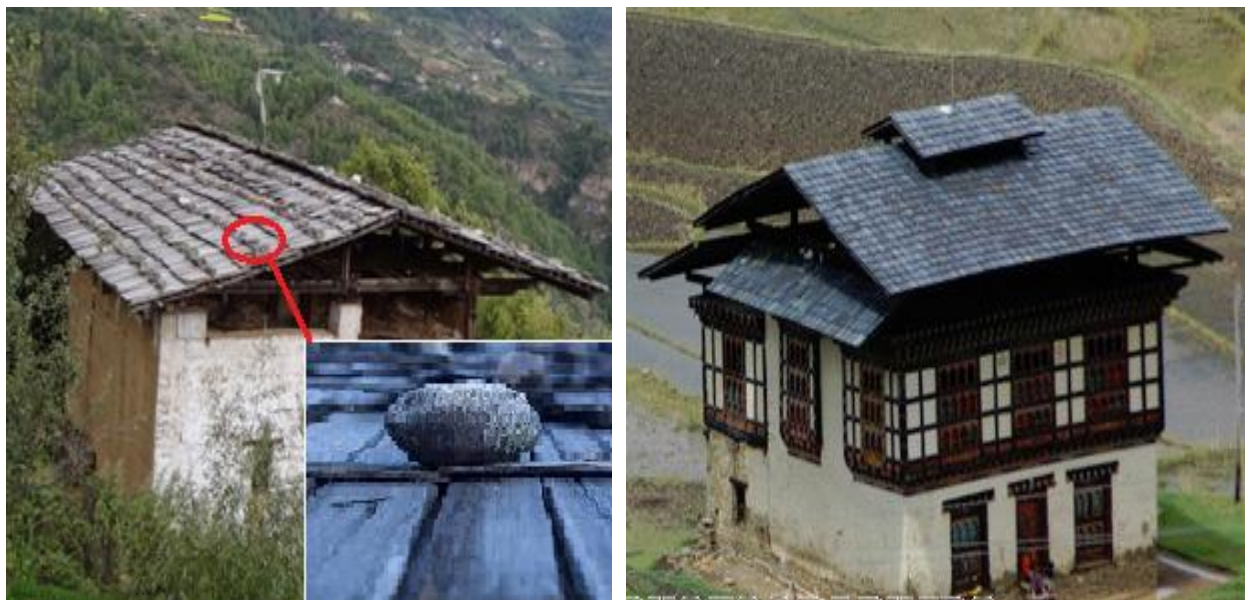
Figure 9 : Wooden shingles (L) and slate roofing (R)
