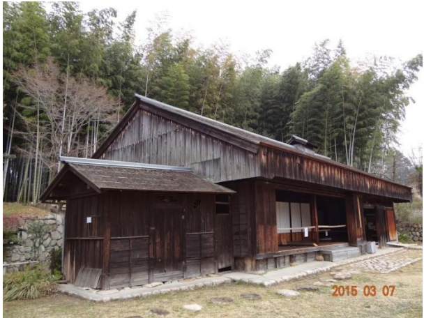
Figure 21 : Gable roof (kirizuma) with thatched roofing (L) and cryptomeria bark roofing (R)
