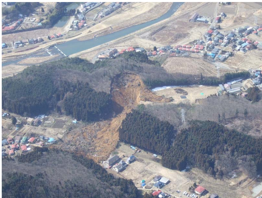
Fig. 80. Tohoku-Taiheiyo Earthquake, Shirakawa, Fukushima (March 2011)
