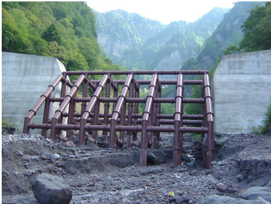
Fig. 116. Open steel pipe in a Sabo dam.
