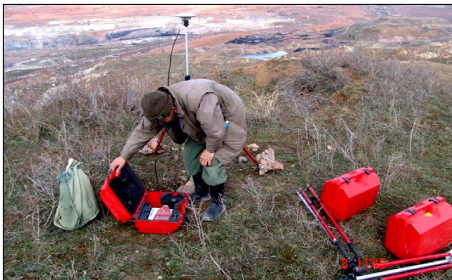
Fig. 67. Electronic tachymeter for shooting landslide.
