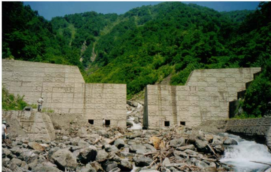
Fig. 118. Concrete-slit Sabo dam before sediment discharge.
