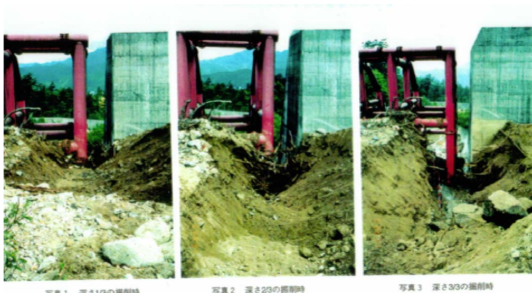
Fig. 117. Grid Sabo dam with trapped debris flow.
