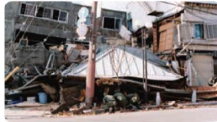
1995: Great Hanshin-Awaji Earthquake; western part of the northern district of JR Shin-Nagata Station (Kobe City)
