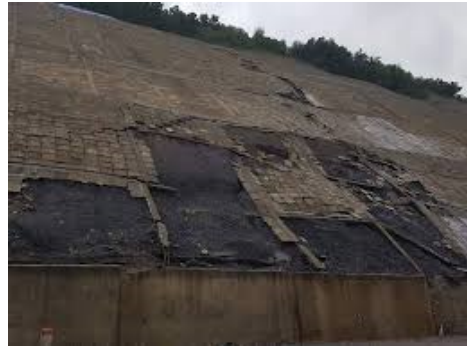
Slope reinforced by concrete slab
