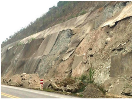
Slope reinforced by concrete mortar
