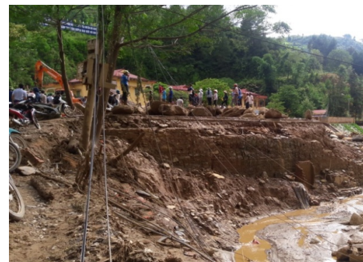
Flash floods and landslide in Mu Cang Chai district, Yen Bai province 2017
