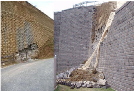
Reinforced by retaining wall
