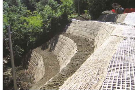
Slope reinforced by Geotextile
