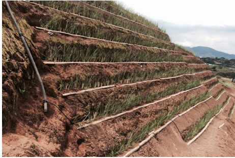
Slope reinforced by Planting vetiver on the slope
