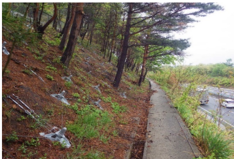
Reinforcement solutions against landslide by metal rock anchor combined with planting tree, grass on the slope
