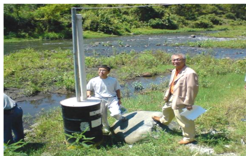
Installation on the concrete basement,( Guatemala)
