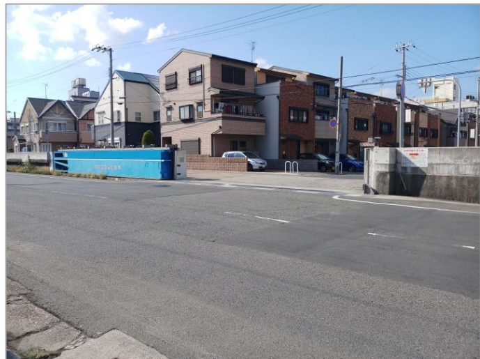
Figure 21: Flood gate at Higashi-nada ward in Kobe
