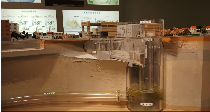
Figure 26: Model showing Kanda River Underground Regulating Reservoir Tunnel
