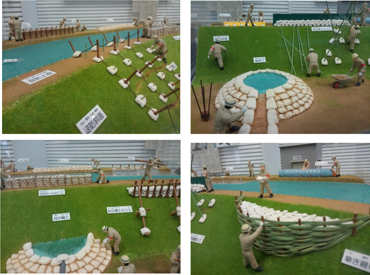
Figure 3: Models showing activities on Flood Protection/ Prevention by Suibo-Dan (Flood Fighters) using sand bags, bamboo and local materials (photo source: Tsunami & Storm Surge Disaster Prevention center, Osaka)
