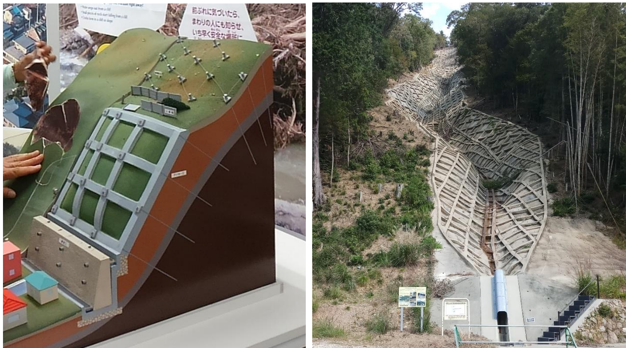
Figure 22 : (A) Model showing Sediment Disaster Prevention using Anchor work in Nigawa Landslide Museum (B) Sediment disaster countermeasures in Tamba city
