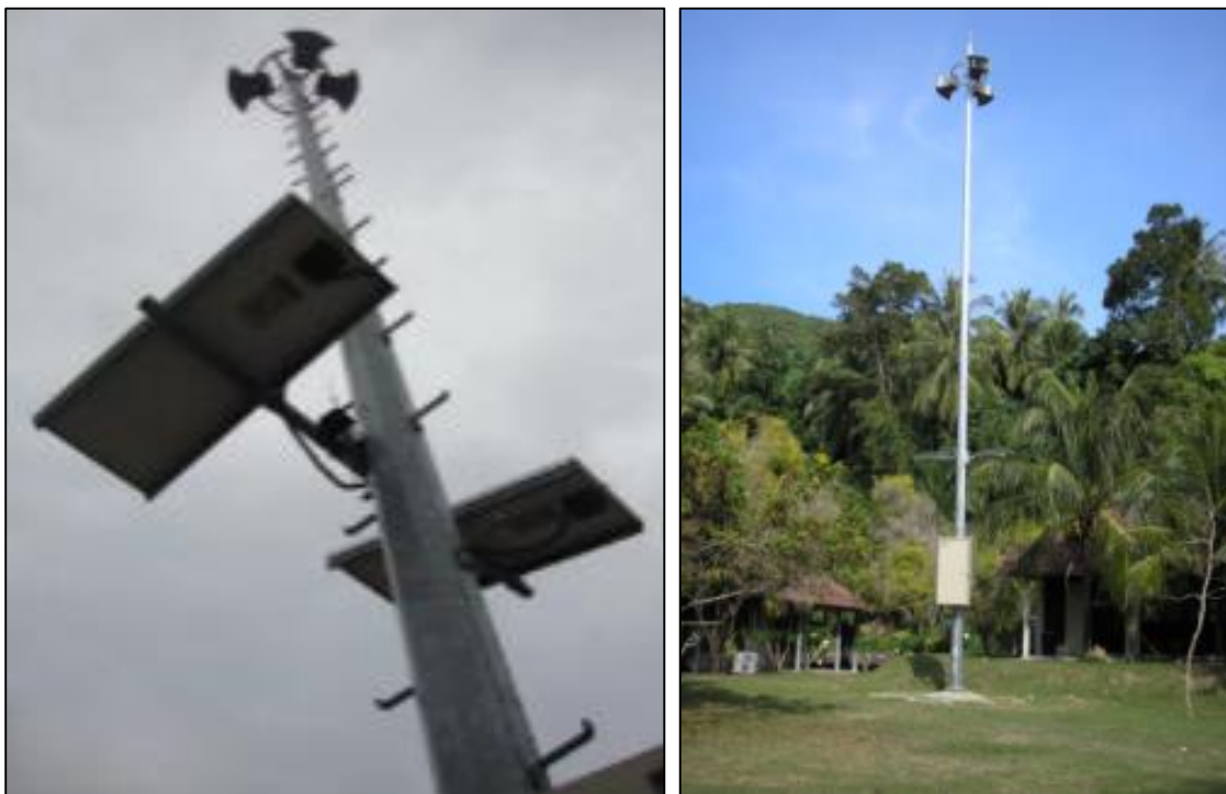
Figure 17: Siren Tsunami Operated by MMD for Tsunami Warning Dissemination
