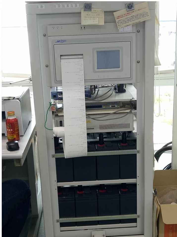
Figure 11: Device for reading Seismic Intensity Meter
