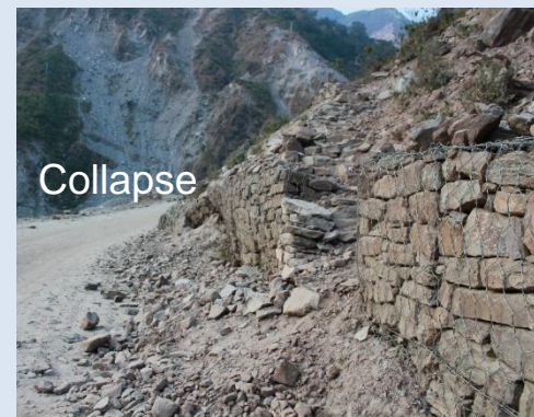
Damage survey on gabion structures along Araniko Highway, Nepal
