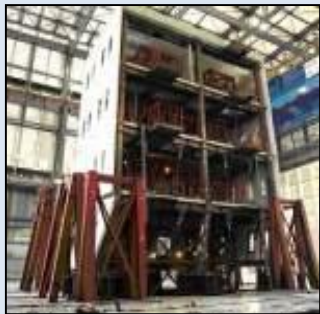
4-story Steel Frame Building
