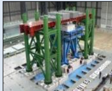
RC Bridge Column constructed in the 1970s
