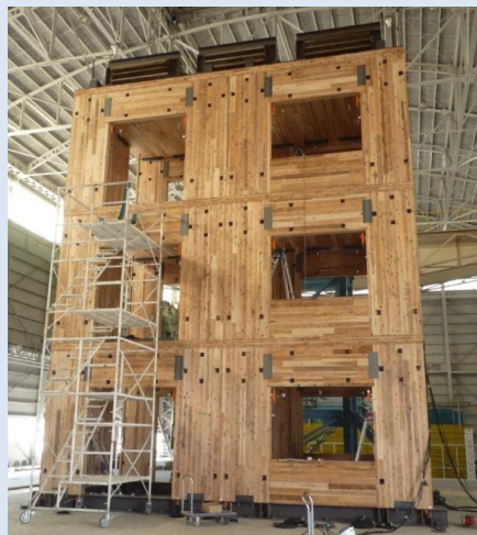
Wood structure built with CLT
