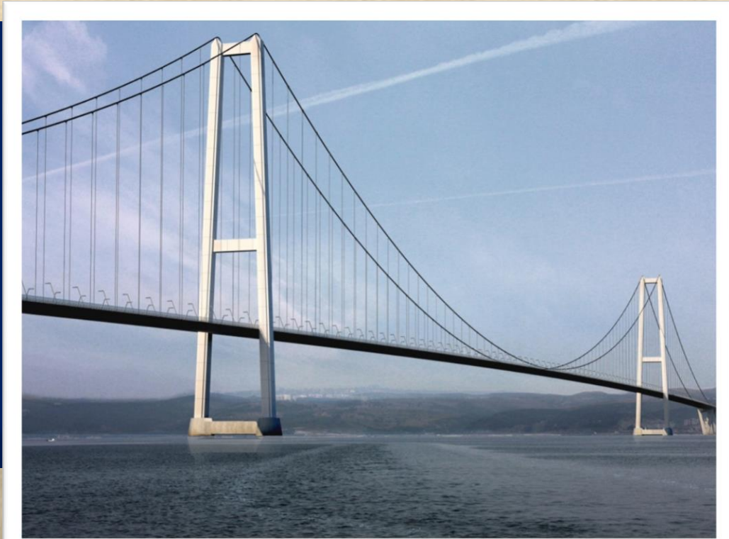
Newest Suspension Bridge Closest to North Anatolian Fault
