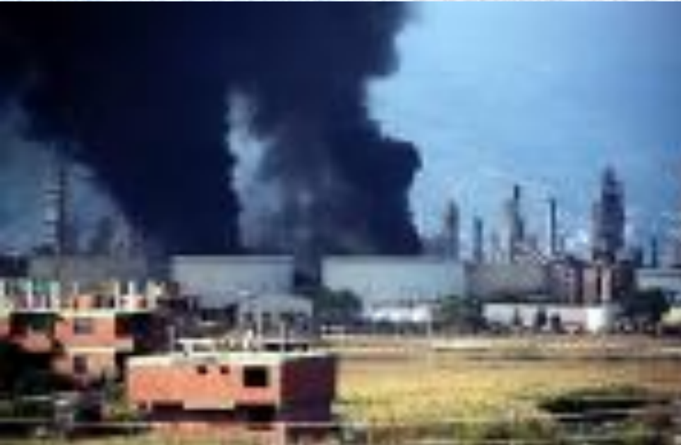
TÜPRAŞ Refinery Fire
