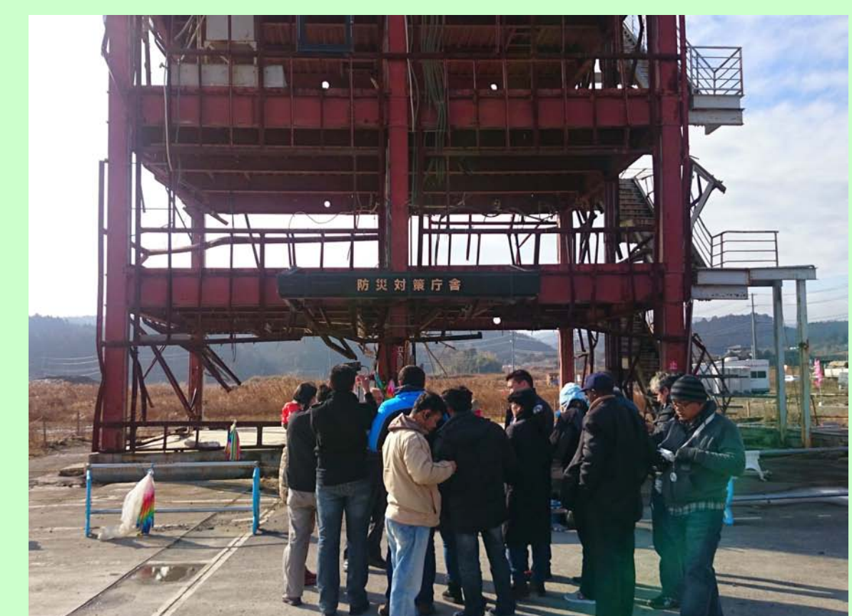
Remains of the Disaster Management Office of Minami Sanriku-cho, Miyagi Prefecture
