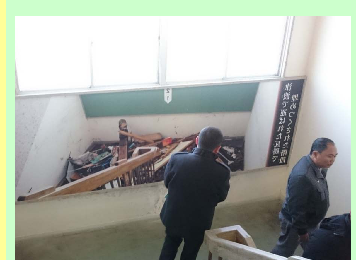
Remains of the Arahama Elementary School, Sendai city, Miyagi Prefecture
