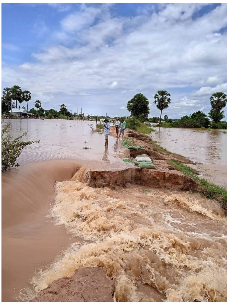
Photo 3: The Access road affected by flood in Kandieng District of Pursat Province in 2025
