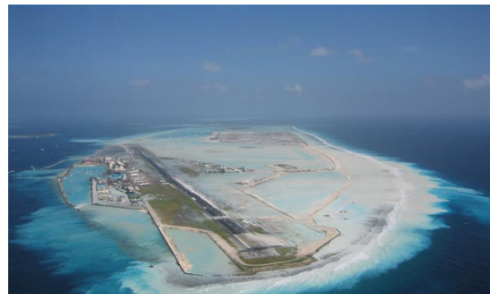
Figure 24: International Airport on tsunami - 2004
