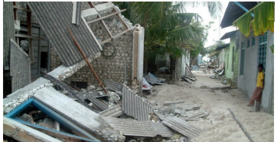
Figure 23: Damages caused due to tsunami - 2004
