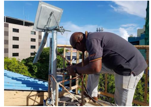
FIGURE 35: ESTABLISHING EW BACK SYSTEM
