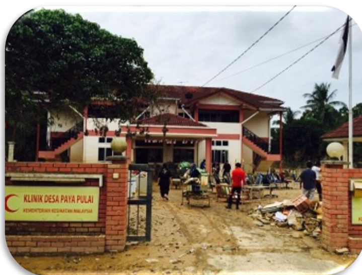
Post Disaster Voluntery Works
