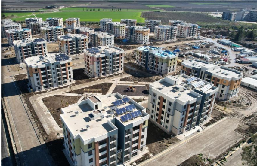
Photograph 17. Newly Built Disaster Housing
