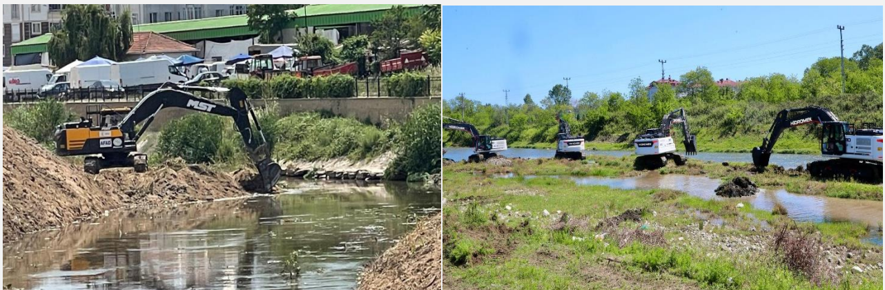
Photograph 14. Stream Improvement Works
