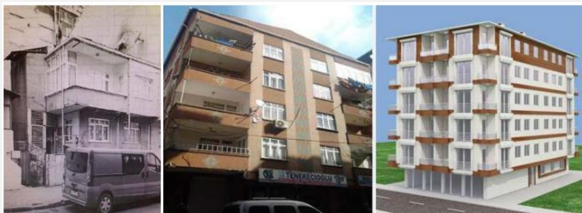
Photograph 15. Transformation of Disaster Risk Structure
