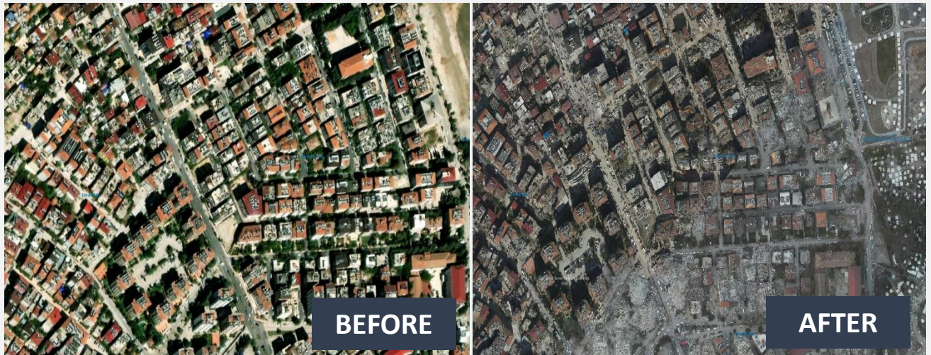
Photograph 9. Kahramanmaraş Earthquake Before and After Images
