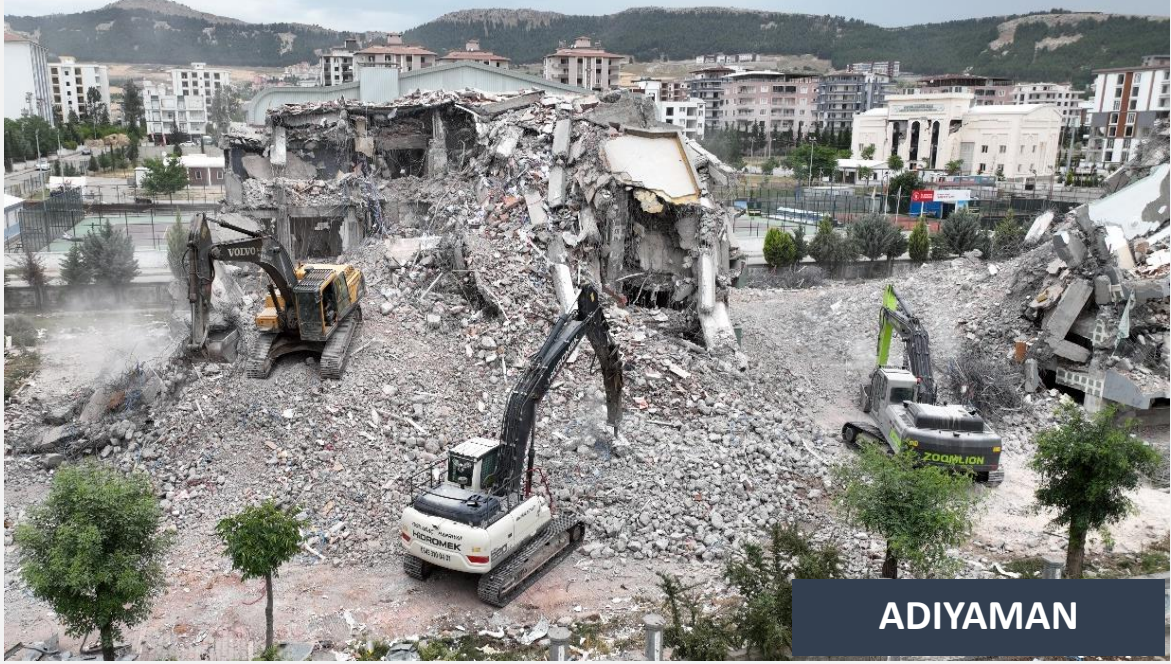
Photograph 8. Debris Removal Work
