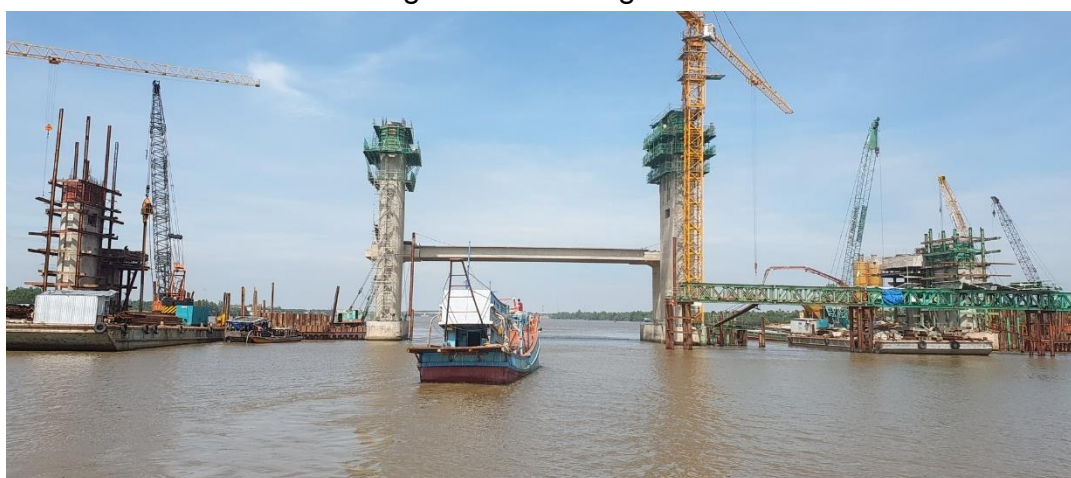
Figure 16 : Cai Lon – Cai Be irrigation system under construction
