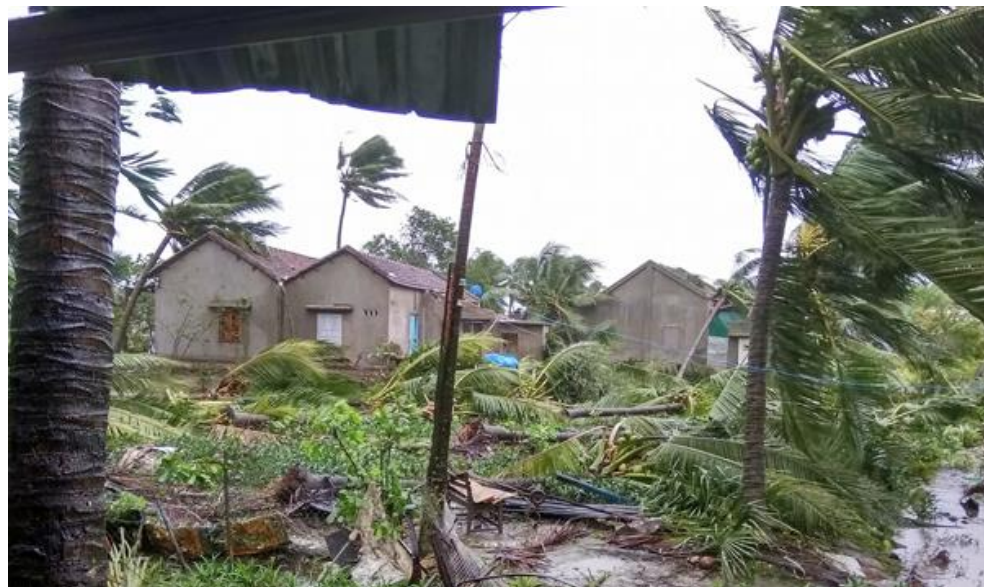
Figure 10: Damages caused by Damrey Typhoon in Khanh Hoa Province
