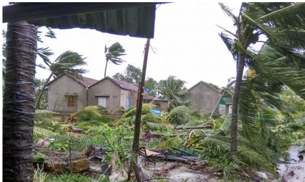
Figure 12: Damages caused by Damrey Typhoon in Khanh Hoa Province
