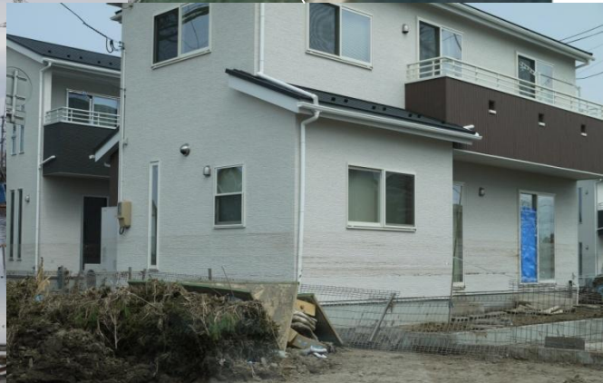
Water level could be 1.5m high
