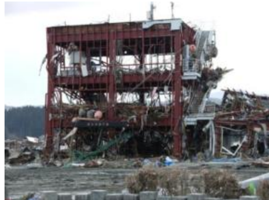
The disaster management center of Minami-Sanriku town(2011.3.23)
