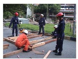
Fig. 4-2-1-2 Temporary column construction training for a collapsed building rescue mission
