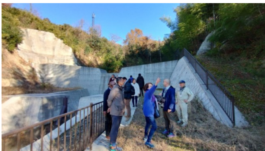
Figure 4.7 Part of the activities during the site visit to Tajimi Sabo National Highway Office
