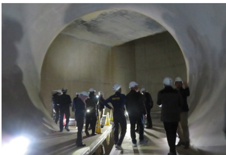
Figure 4.10 Site visit to flood countermeasure infrastructure
