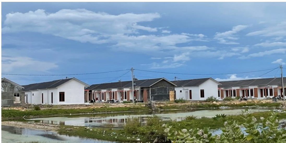
Figure 2.11 New houses built near the coast in Banda Aceh
