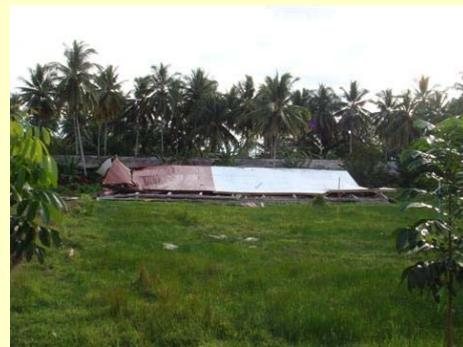
Totally destroyed junior high school building with roofs made of a light material- corrugated tinplate- and limited number of thin pillars
