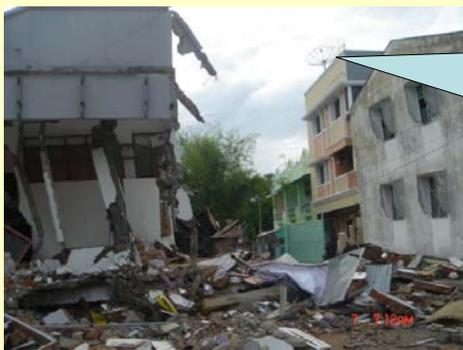
Commercial building with the first floor crushed
