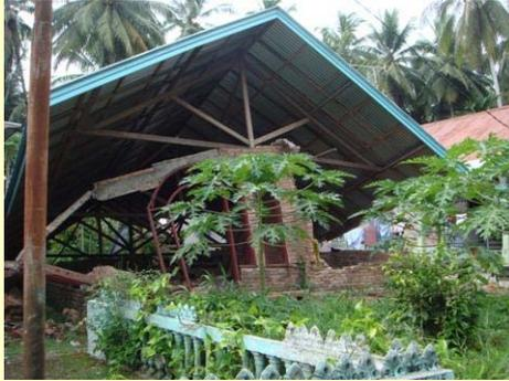
Destroyed building due to the collapses of brick walls
