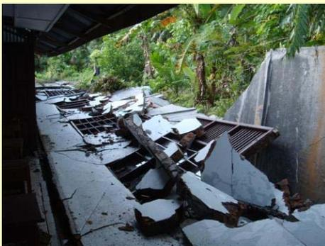
Collapsed junior high school' s wall with pillars and beams reinforced by steels but the steels are found not connected properly.
